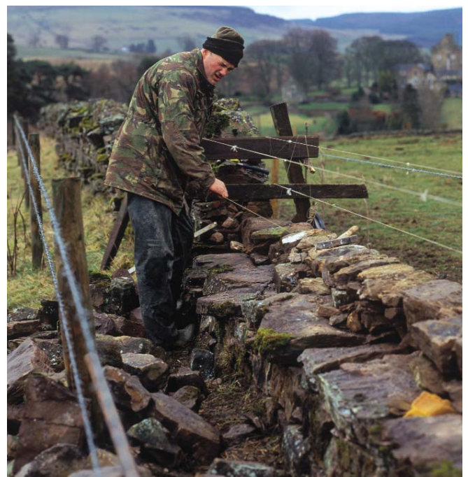
Photo: Repairing a dry stone wall near Elsdon
