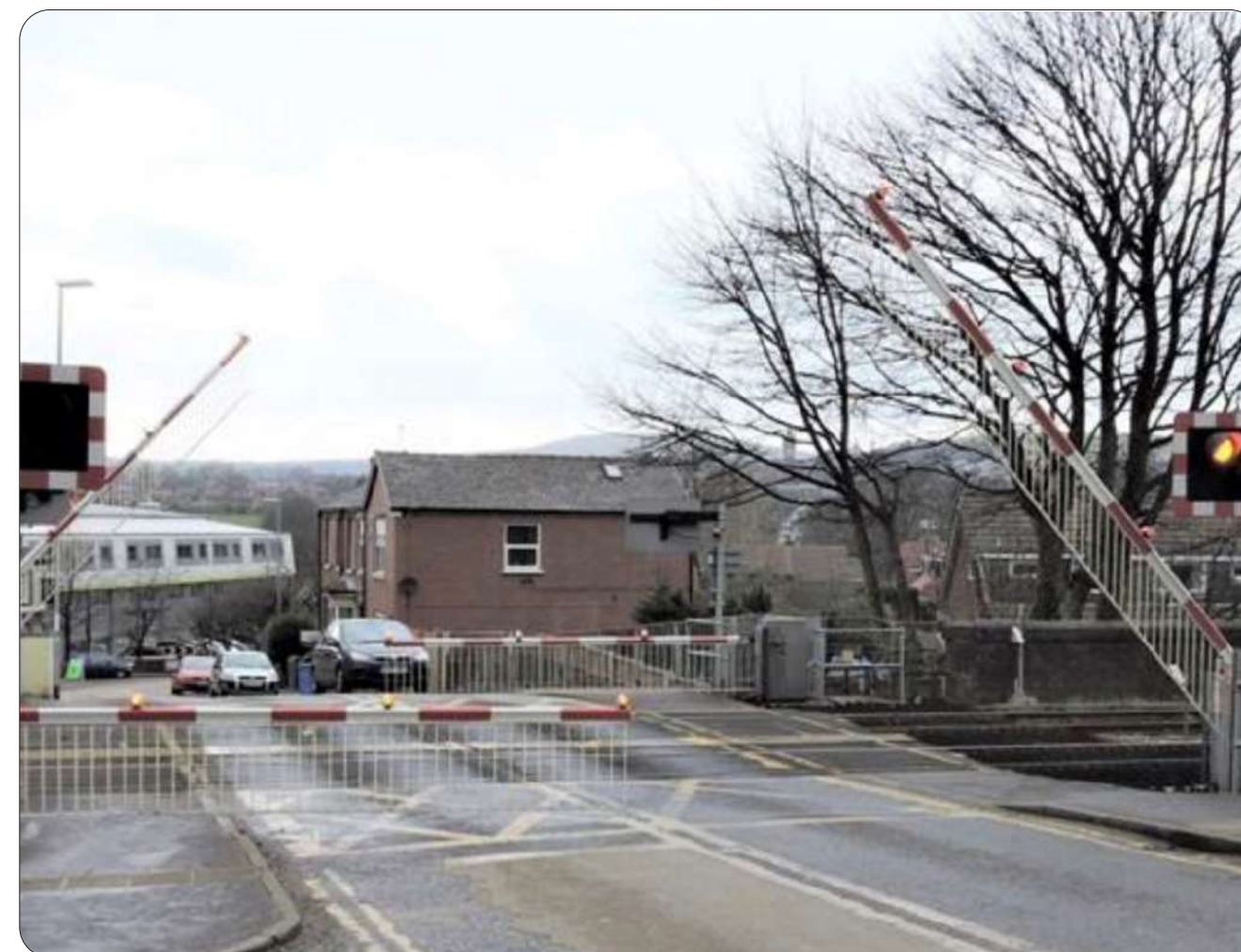
Figure 7: Example of the type of level crossing proposed for Green Lane
