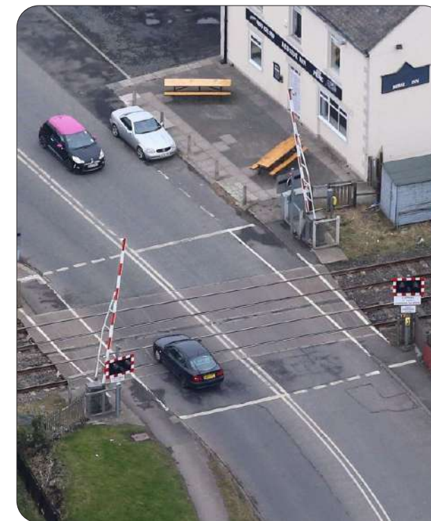
Figure 18: Bebside level crossing as it is today
