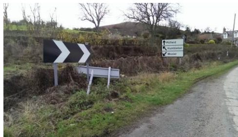
Photograph 15: View showing damaged Chevron Boards and Northbound stack type sign
