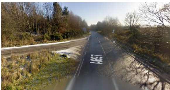
Photograph 3: View showing southbound approach to layby
