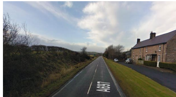
Photograph 10: View heading Northbound adjacent to Station Cottages
