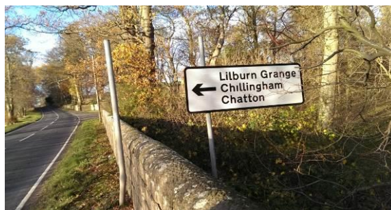
Photograph 18: View showing ADS facing wrong direction detached from pole
