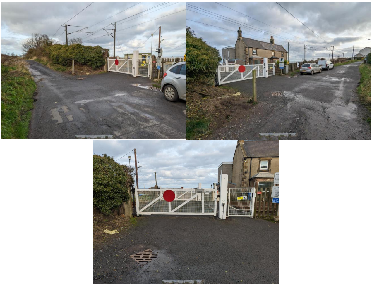
Photographs of the Cow Road crossing point.
