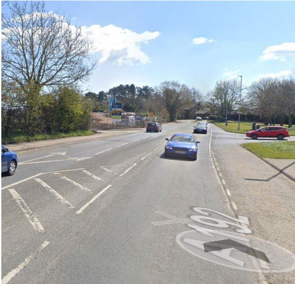
A192 Pottery Bank Morpeth – Southbound Approaching the New Development (on the left)
