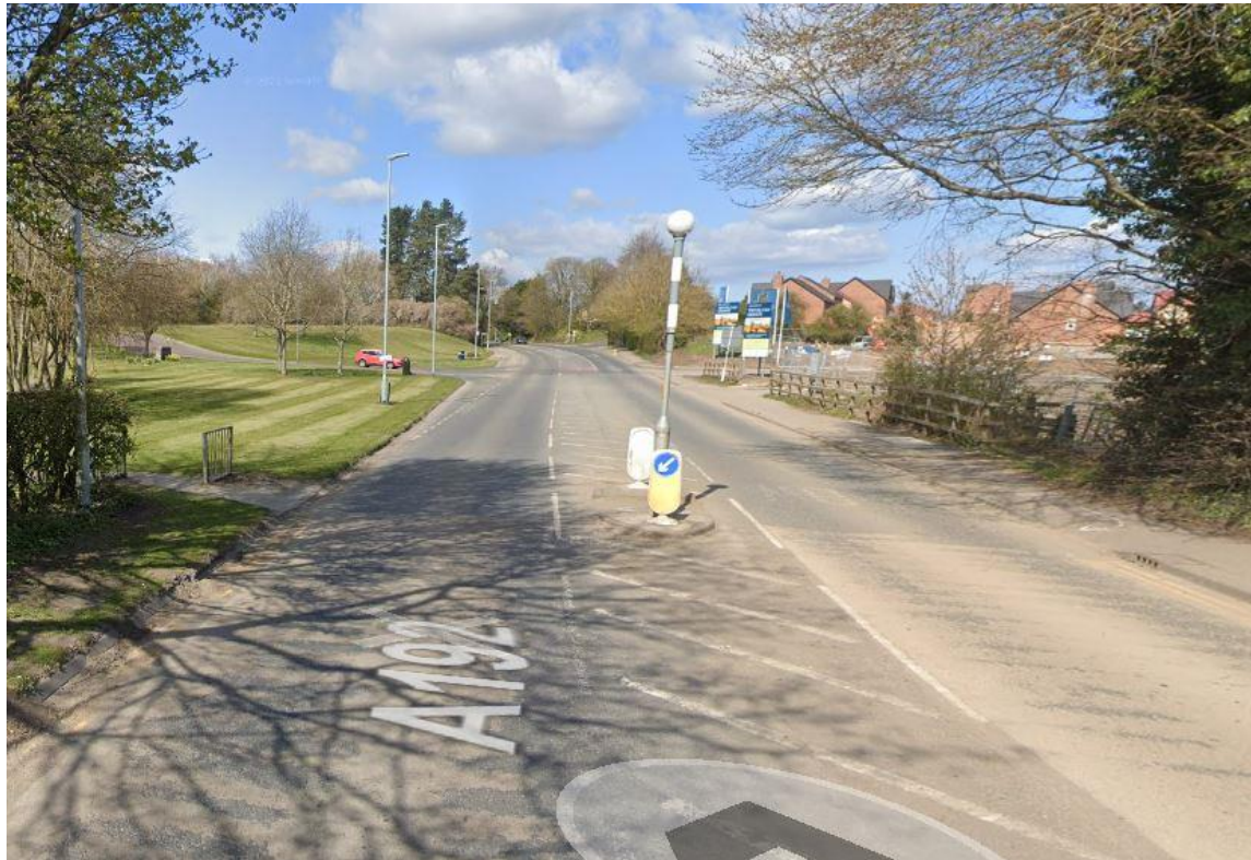
A192 Pottery Bank Morpeth – Northbound Approaching the New Development (on the right)
