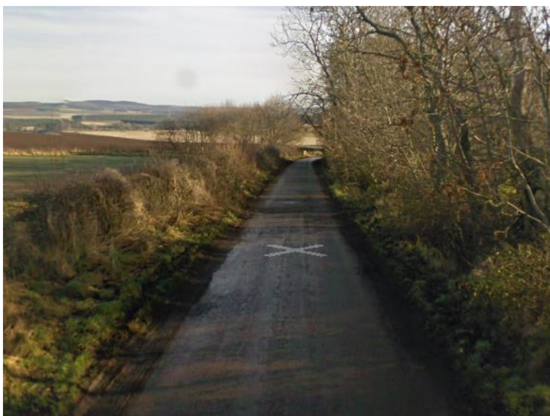
Fig.3. A section of the road west of Milfield Hill, looking south east.
