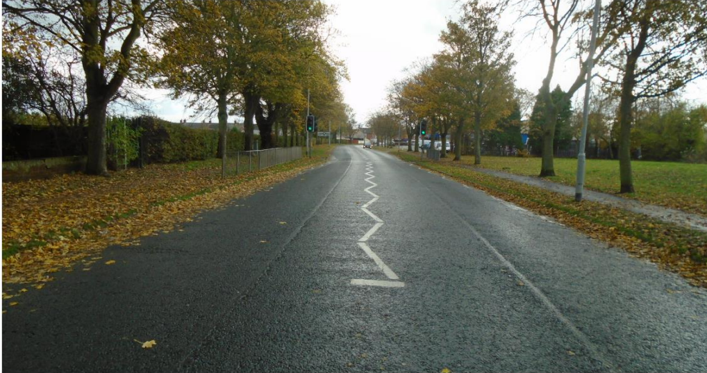
Figure 2 – Existing layout of North Seaton Road, Ashington (southbound approaching Newbiggin Road)
