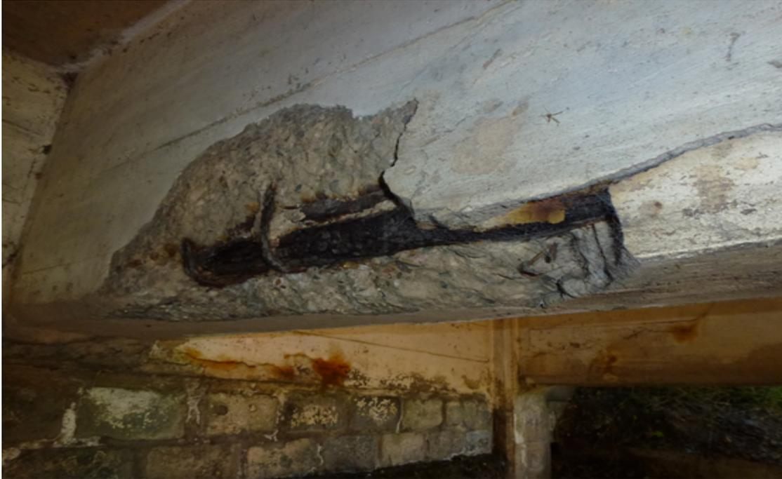
Deck soffit detail showing longitudinal cracking to base of main and secondary RC beams. Also note leachate staining and stalactite formation
