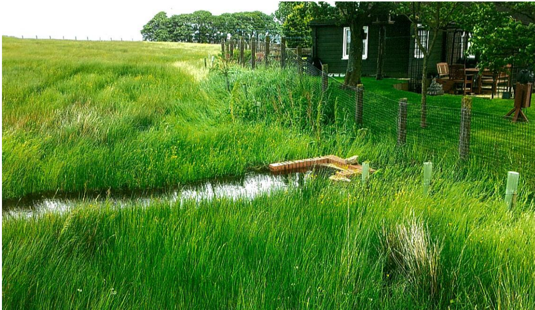
Figure 1: The blocked inlet west of Leaside, Halton Lea Gate
