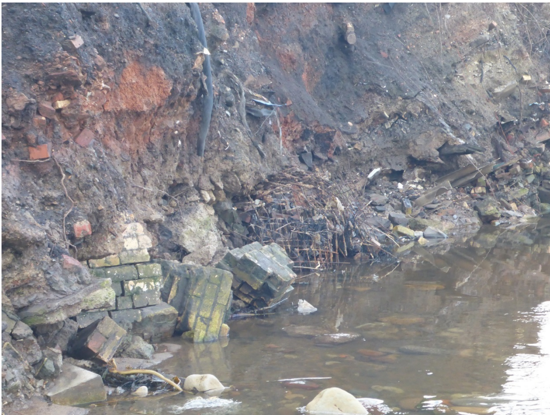
Plate 2 – Hot spot #1 - Erosion of brickwork, construction rubble, metalwork and rubber tubing from the colliery spoil river bank at the mouth of the River Lyne
