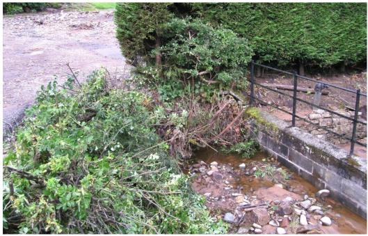
Figure 2: Debris and the blockage of a culvert in Bankfoot post 28th June
