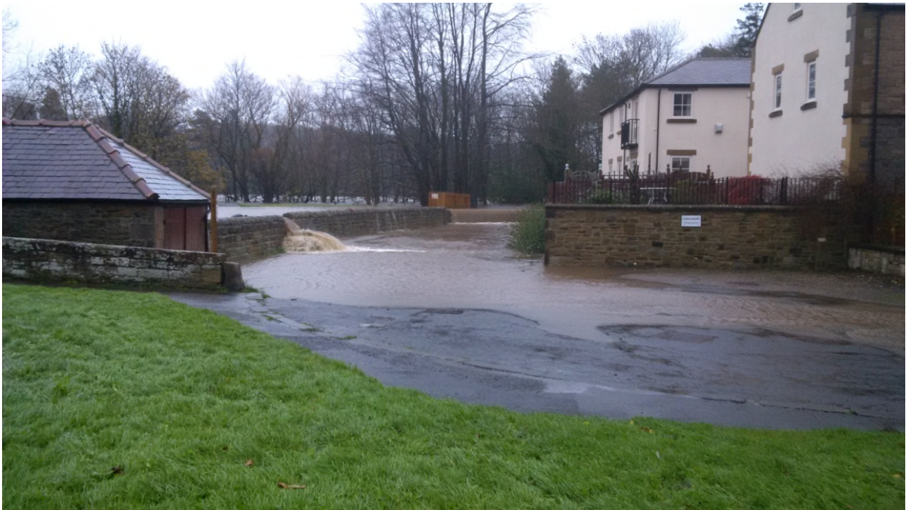
Flood wall overtopping at The Stanners, Corbridge on 5 th December 2015
