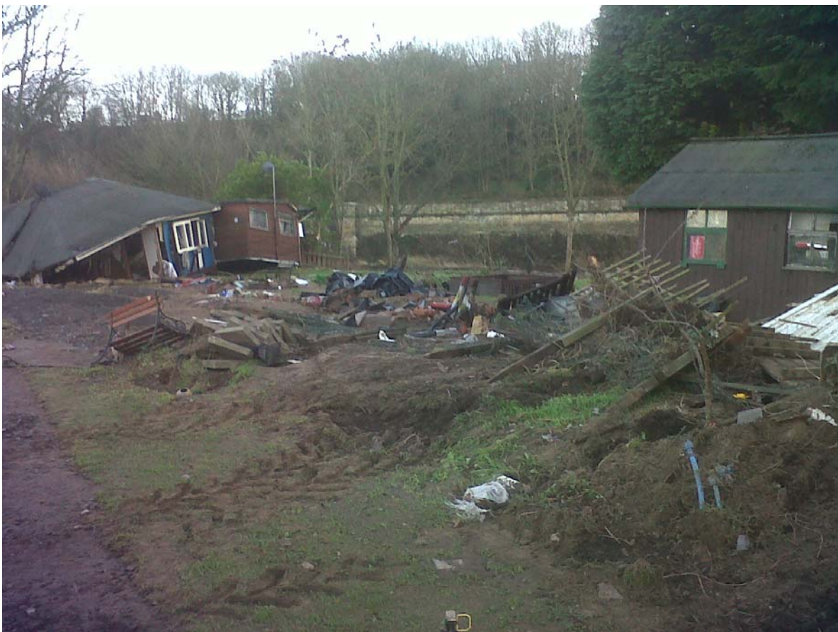
Flood damage at Ferry Landing Holiday Park, Ovingham following Storm Desmond
