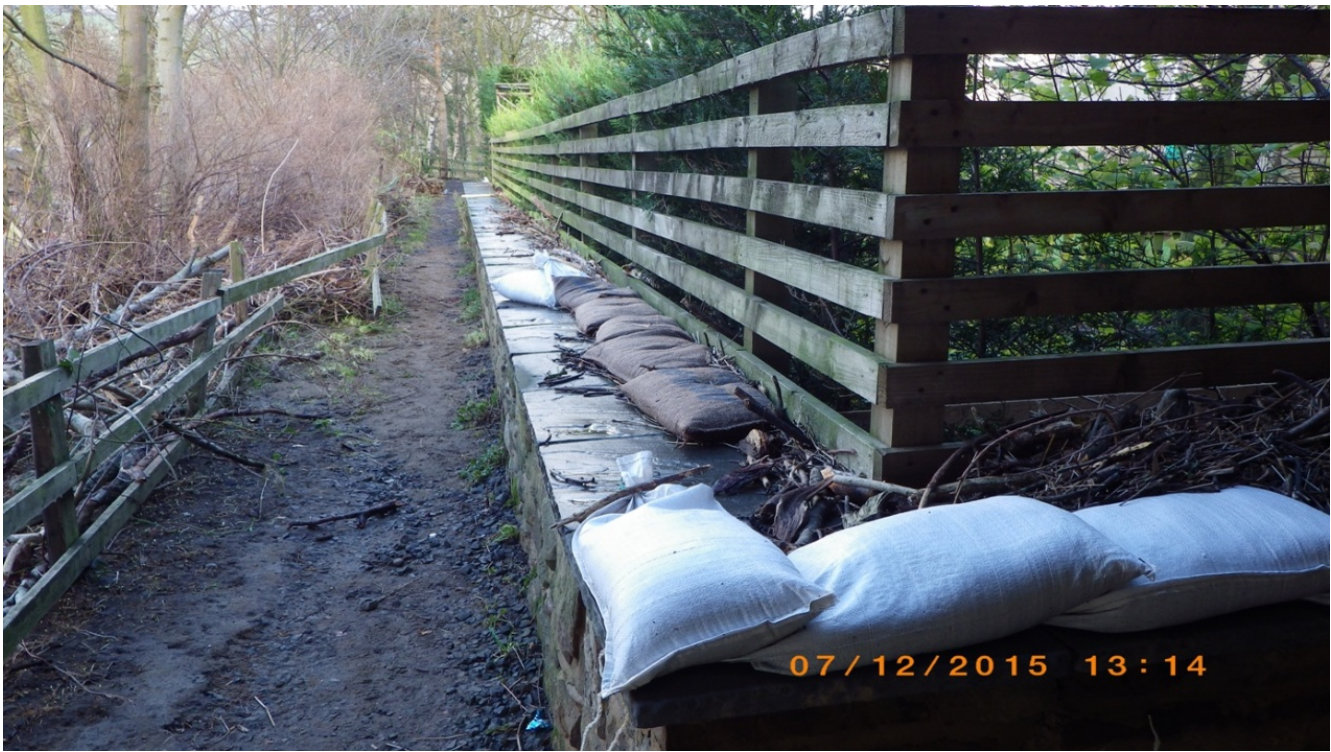
Overtopped flood defence protecting the Temple Houses area of Haydon Bridge in the aftermath of Storm Desmond
