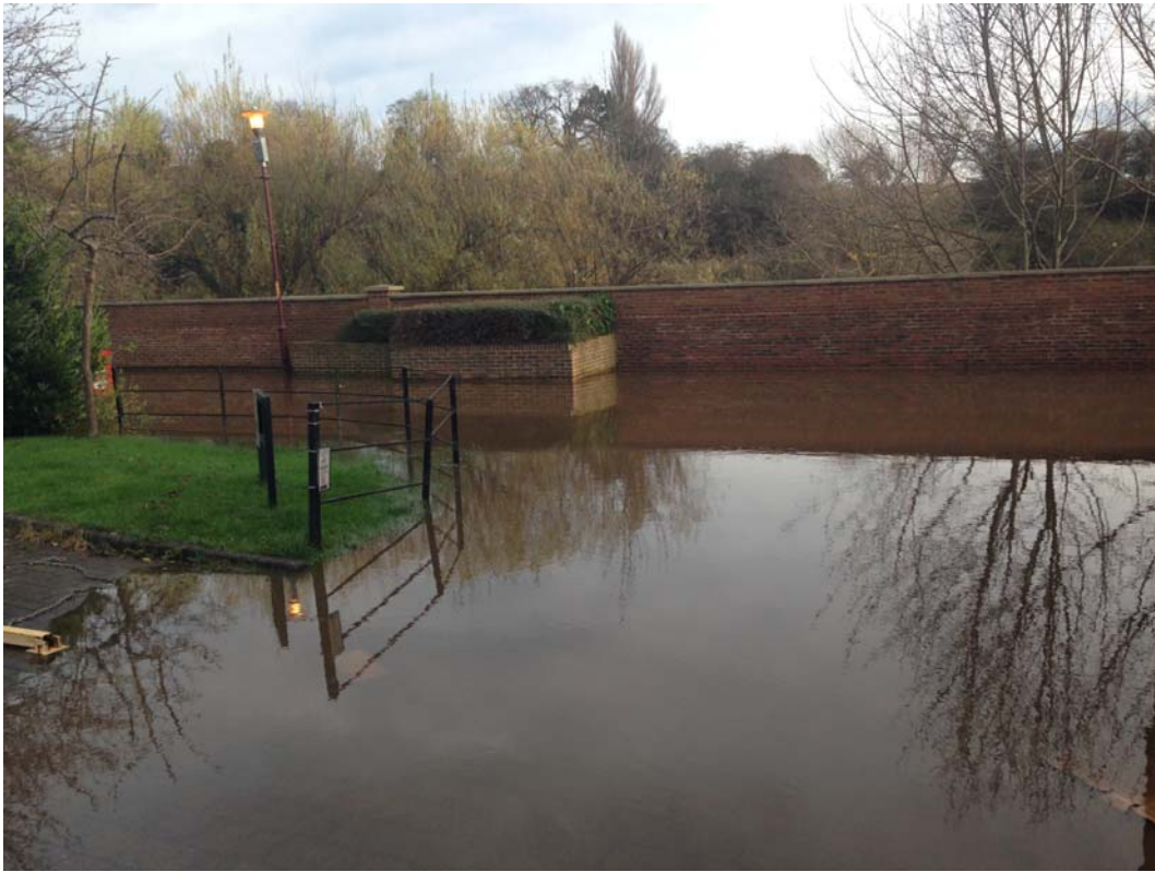
Surface Water Accumulations on dry side of flood wall - Yarm
