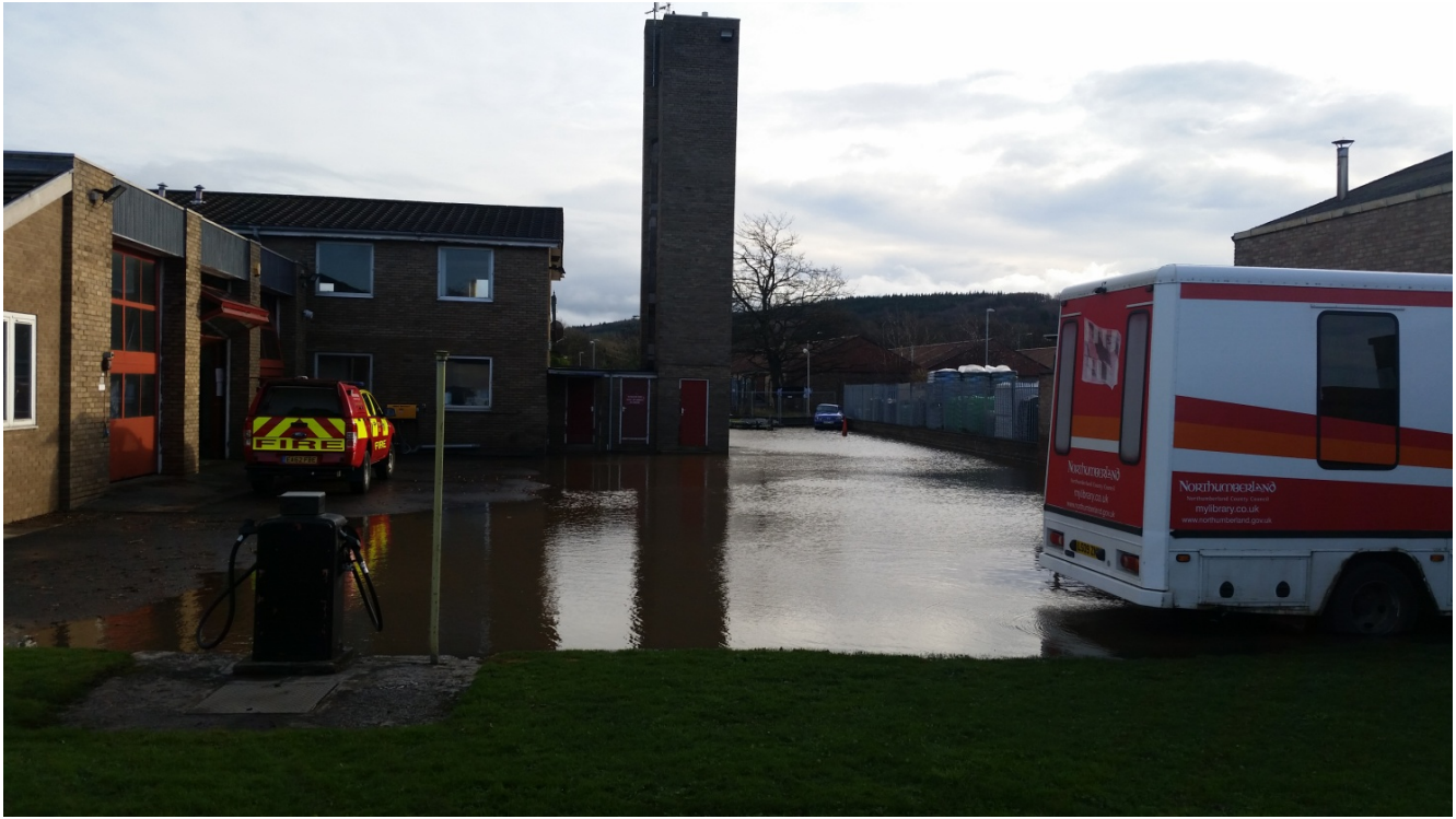
Flooding at Tyne Mills Industrial Estate, Hexham on 5 th December 2015
