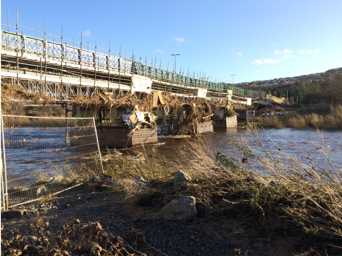
Flood damaged scaffolding at Ovingham Bridge following Storm Desmond
