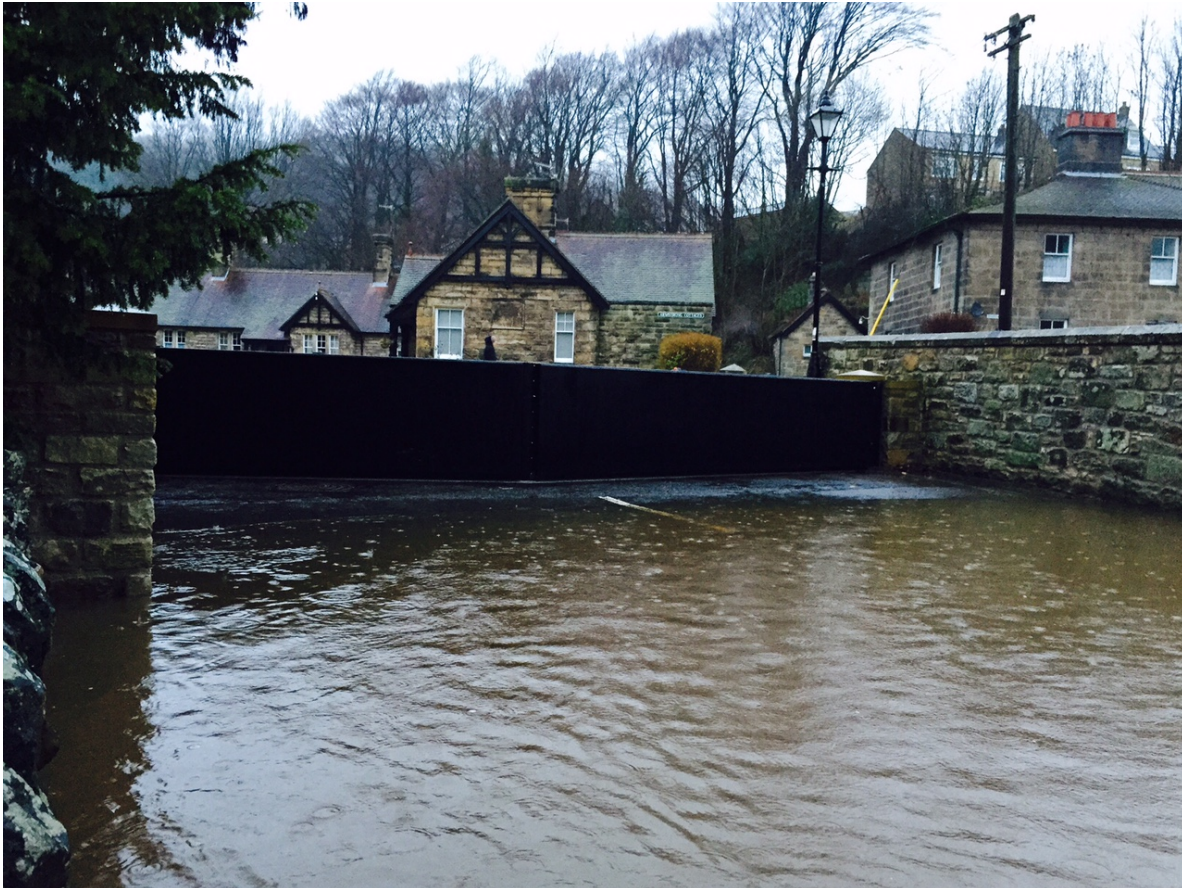
Floodwater behind our floodgate at Rothbury during Storm Eva on 26 th December 2015
