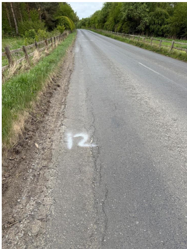
Hotbox Patching Before C03 C342 Matfen to B6318
