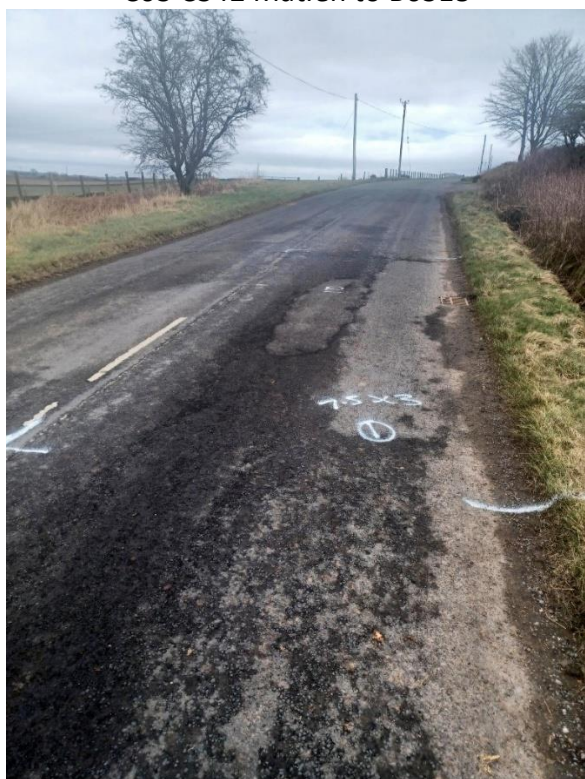
Hotbox Patching Before C03 C342 Matfen to B6318
