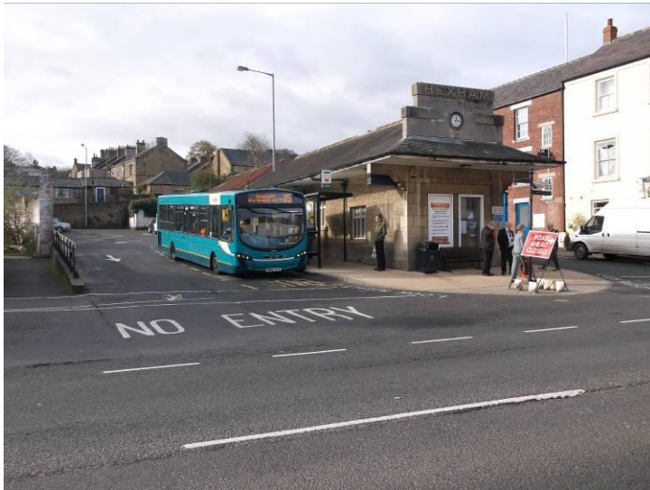
Photograph 1 - Existing Bus Station
