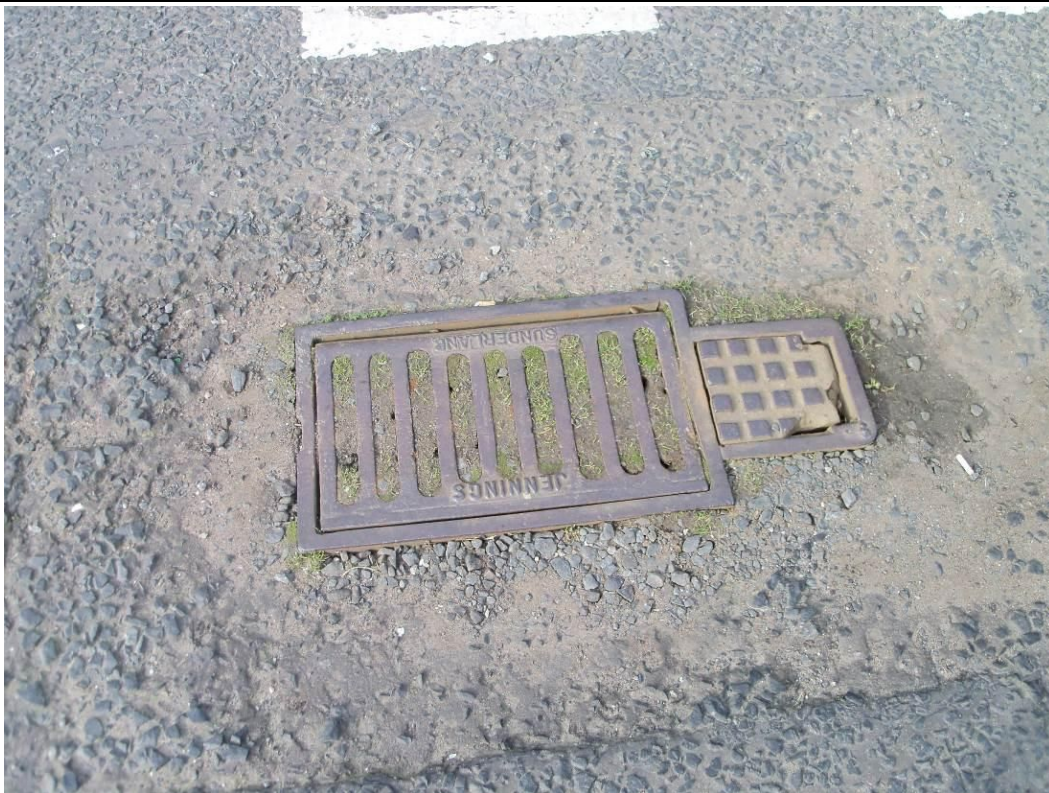
Photograph 6 – blocked surface drains
