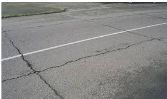
Reflective cracking
