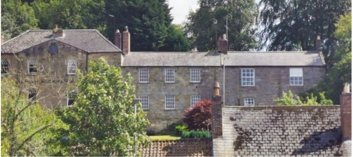
Figure 4: Chimneys, materials, window styles and roofscapes all contribute to quality of design – Roofscape in West Thirston
