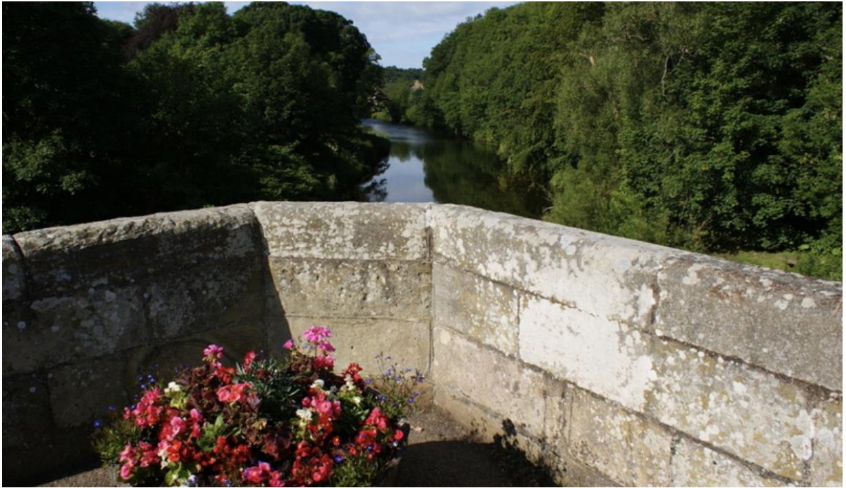
Figure 6: River Coquet SSSI as seen from the pedestrian bridge (a scheduled monument)
