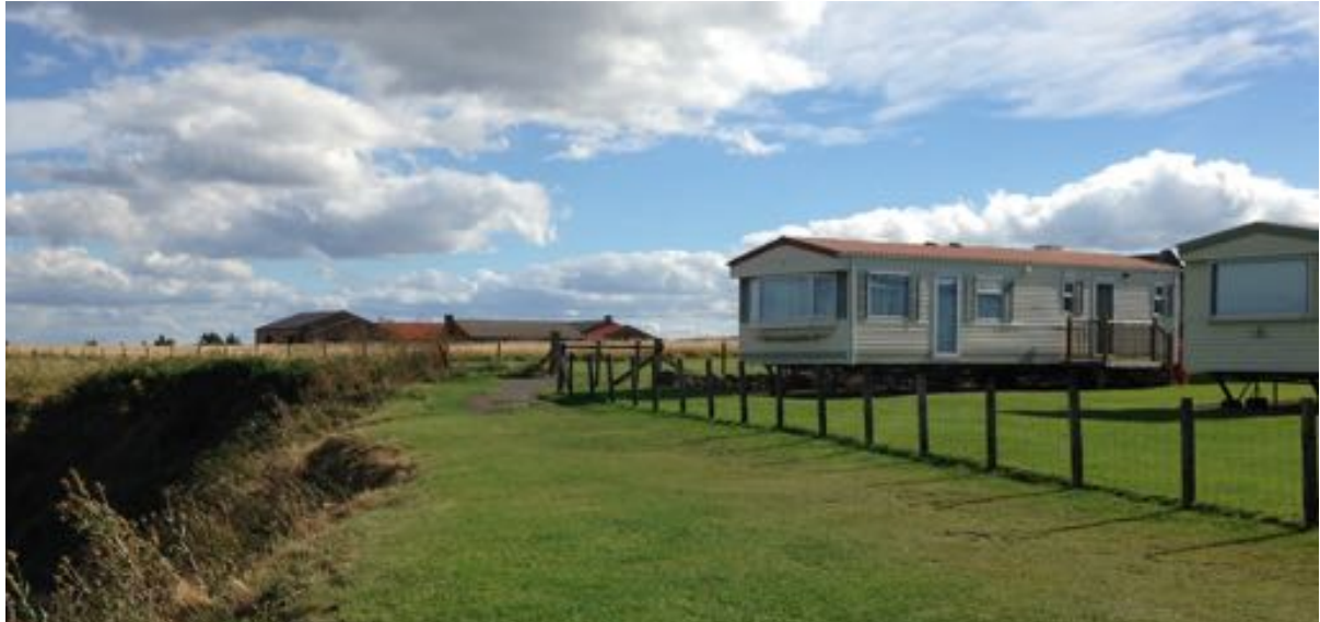
Photo 3: Caravan park in Seahouses - fenceline forms settlement boundary. Sewage works visible in background - field excluded
