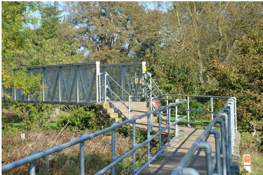
Photograph 7: Steppey Lane footbridge
