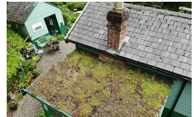
Figure 104: Good example of green roof, The Garden Station at Langley
