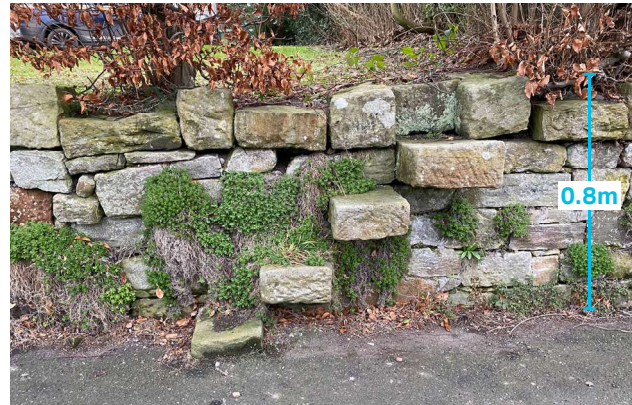
Figure 53: Mounting steps with squared crenellation coping, Eglingham
