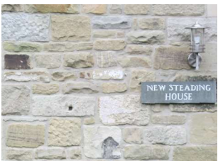
Mortar tone matches sandstone
