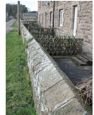
Figure 55: Saddle (pointed) coping stones, North Charlton
