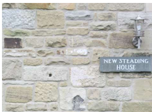
Mortar tone matches sandstone
