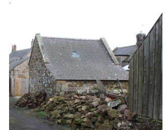
Water tabling on outbuilding
