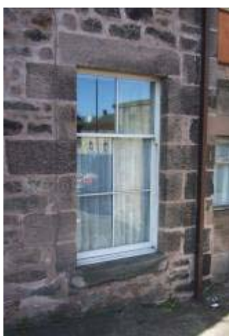
Larger square dressing stones to rubble wall; raised dressings to coursed wall; rounded corner details
