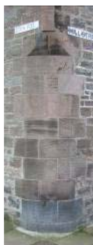
Larger square dressing stones to rubble wall; raised dressings to coursed wall; rounded corner details
