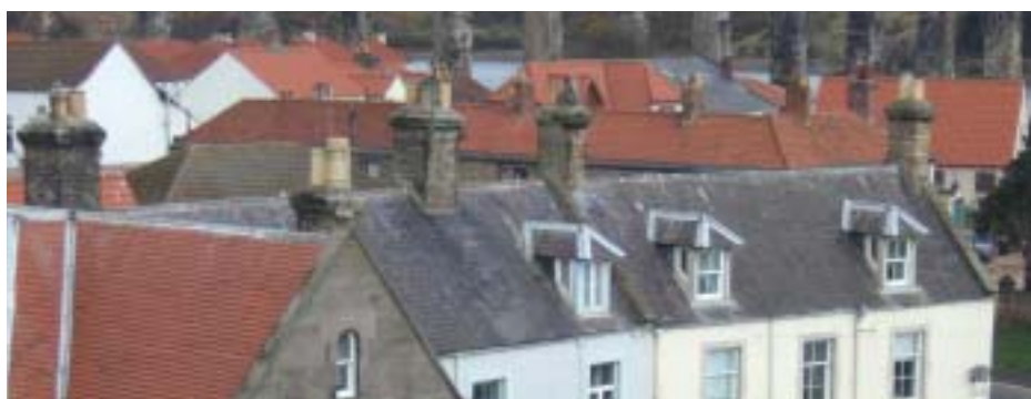
Natural slate (right bottom) and clay pantiles (right top) provide a vigorous, spirited scene from above
