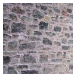
Local sandstone – rubble, square coursed blocks, and (less common here) ashlar
