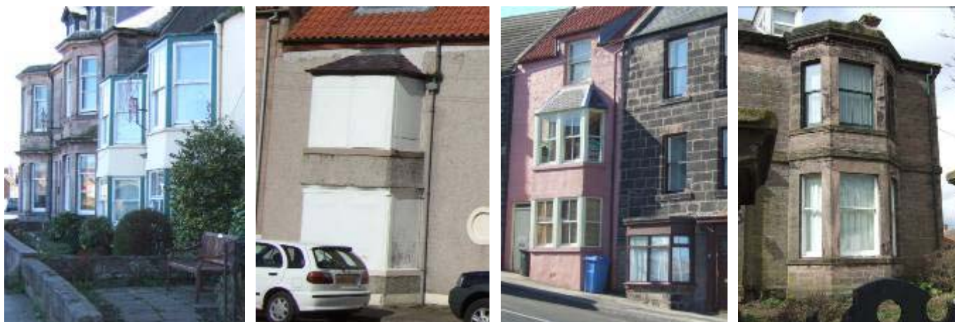
Above: angled bay windows in stone and timber, Main Street, West End, Kiln Hill, Main Street. Below: bow windows and modern oriel bay
