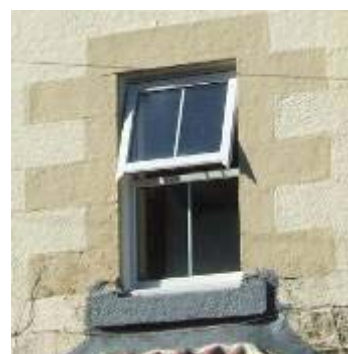
Windows and doors in particular suffer inappropriate alterations which harm architectural and historic character
