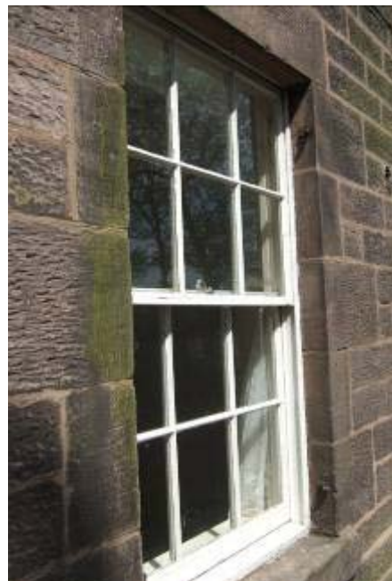
Traditional timber vertical sliding sash windows, set back into a reveal
