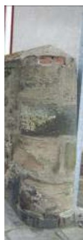
Larger square dressing stones to rubble wall; raised dressings to coursed wall; rounded corner details
