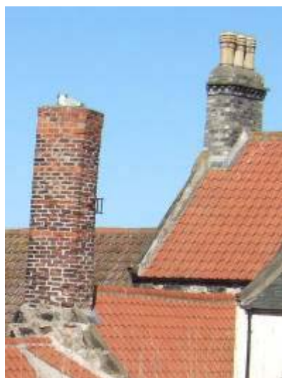
Older brick chimneys often have large dimensions and twists to reveal their age
