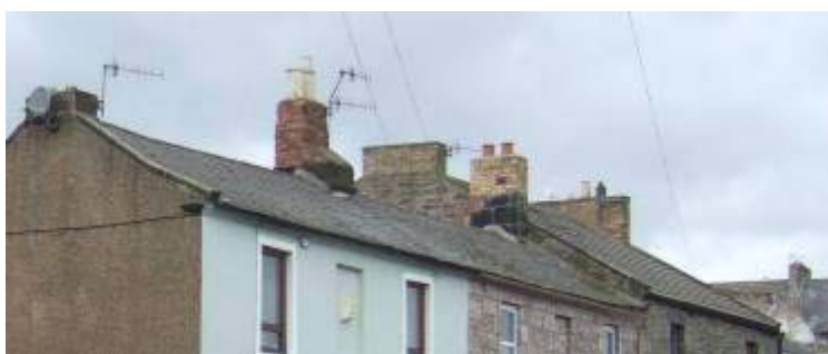
Dropped, capped and shortened chimneys blunt the roofscape. Many have been rebuilt in non-matching materials, whilst others are rendered or over-pointed
