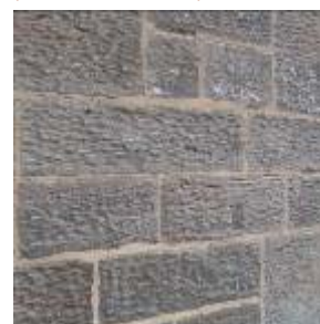
Local sandstone – rubble, square coursed blocks, and (less common here) ashlar
