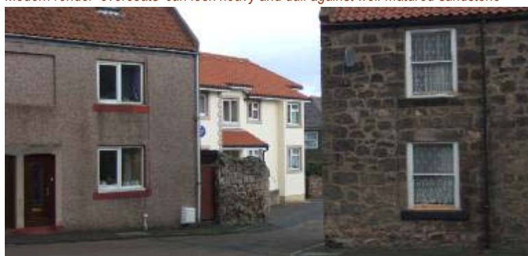
Modern render 'overcoats' can look heavy and dull against well-matured sandstone
