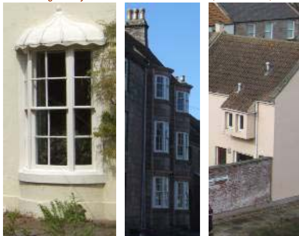
Above: angled bay windows in stone and timber, Main Street, West End, Kiln Hill, Main Street. Below: bow windows and modern oriel bay
