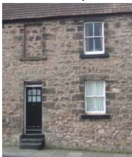
Sandstone masonry, Main Street
