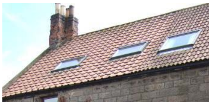
Large modern rooflights should be avoided on front and prominent rear slopes
