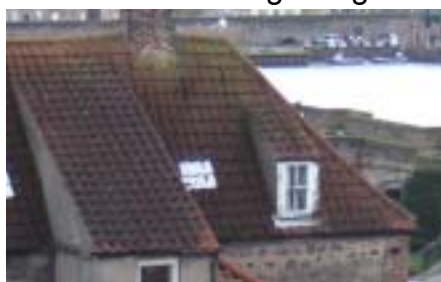
Early catslide dormer, Main Street, and latter Victorian dormers with dual pitched roofs and glazed cheeks
