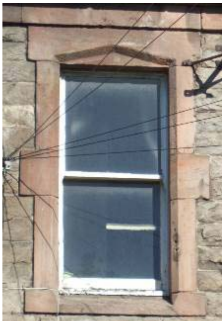
Traditional timber vertical sliding sash windows, set back into a reveal
