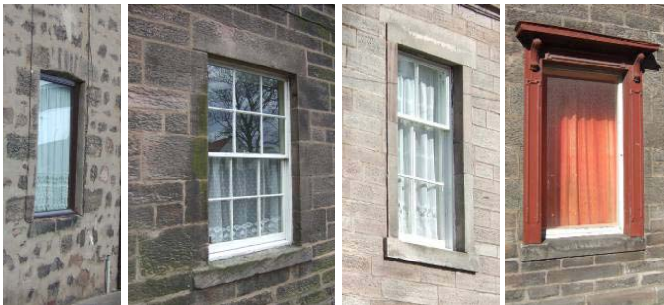
Levels of window emphasis: relieving arch (Blakewell Rd); dressed stones (Church Rd); raised surround (West end); applied timber surround (Main St)
