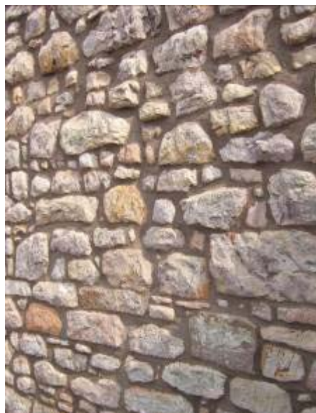
Good work could be better. Left: Good pointing method but a poor mix with insufficient lime. Right: Good match in terms of bonding and stone size, but yellow sandstone is the wrong colour for this area.
