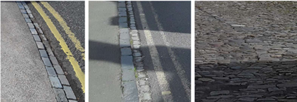
Traditional highway and floorscape surfaces are present, but rare in the conservation area. From left to right: Scoria setts, stone kerbs with setted channel, setted yard.
