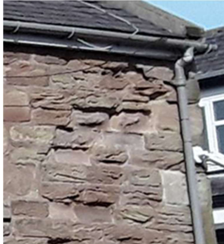
Figure 6.3: Loss and replacement of architectural details
