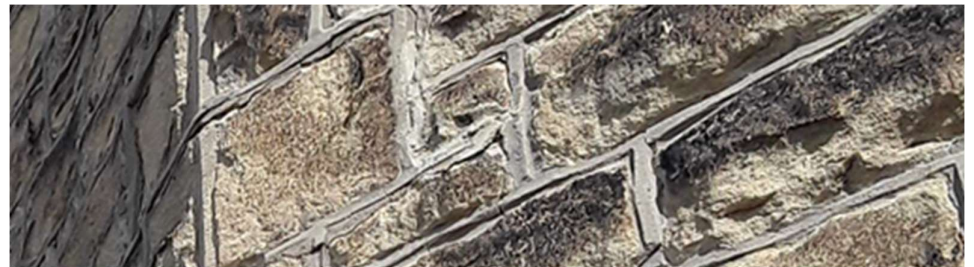
Figure 6.1: Inappropriate mortar and pointing
