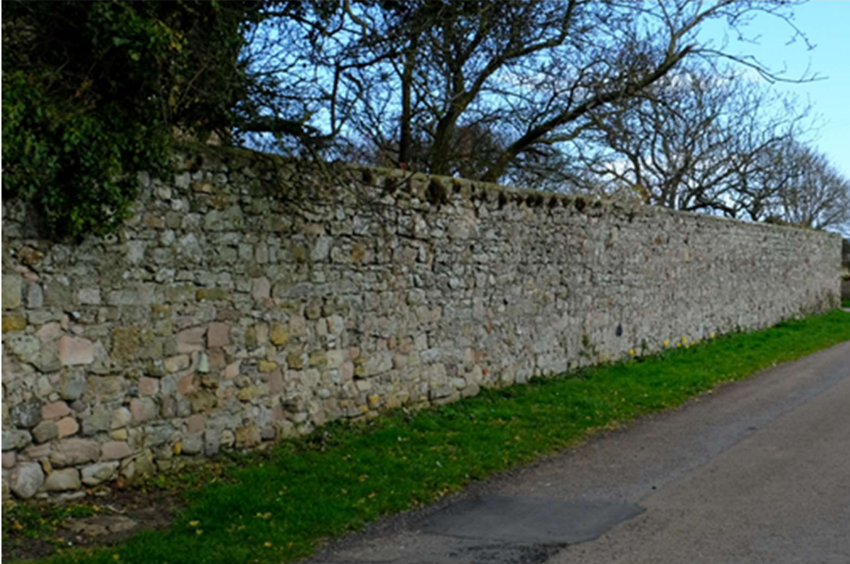
Figure 3.1: Boundary wall made of local sandstone
