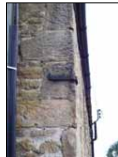
Figure 26 Surviving gate support pin
