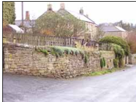
Figure 41 North side retaining wall
