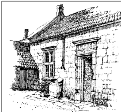
South elevation of Old Manor House, 1890's (originally 2-storey) from Dixon.
