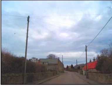
Obtrusive overhead wires and poles
