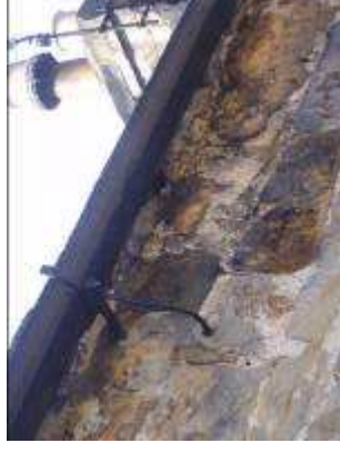
Traditional spiked iron gutter South Cottage
