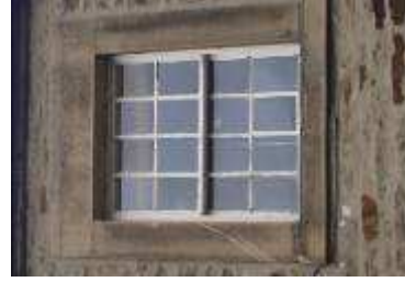
Traditional timber sliding sash window, Red Lion
