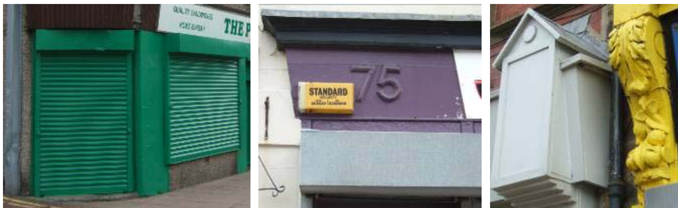
Above: Later additions can harm the appearance of traditional shopfronts. Corbels must be expertly designed and crafted or they will look clumsy against originals. Below: Many shopfronts are altered, with unsympathetic designs and materials, weak detailing, and visual scarring. Bottom: Deep, wide plastic fascia signs unnecessarily dominate the street scene in several places.
