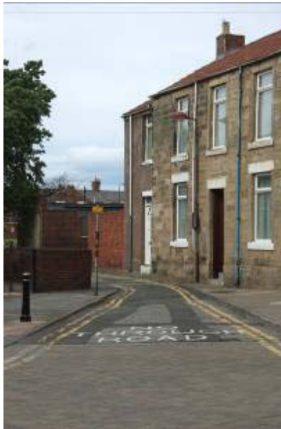
Black tarmac, concrete flags kerbs, scoria block gulleys (far right) and relatively unobtrusive road markings and speed camera.
