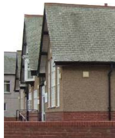
Left: original smooth 1930s render (Café Riviera). Right: original roughcast render above brick plinth (Library, Gibson Street).
