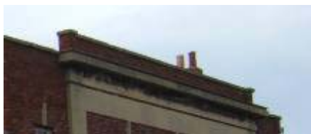
Most eaves are plain but some have simple cornices Bottom: the parapet to No.116 Front Street.
