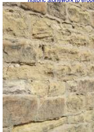
Render and masonry paint dull the scene compared with mature brick and stone. Cement pointing causes historic stonework to erode
