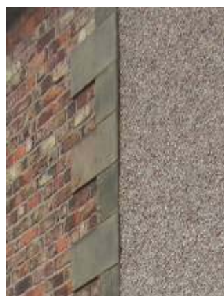
Render and masonry paint dull the scene compared with mature brick and stone. Cement pointing causes historic stonework to erode
