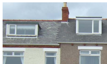
Roofscape can be harmed by modern materials, poorly designed and sited dormers and rooflights, and loss of chimneys
