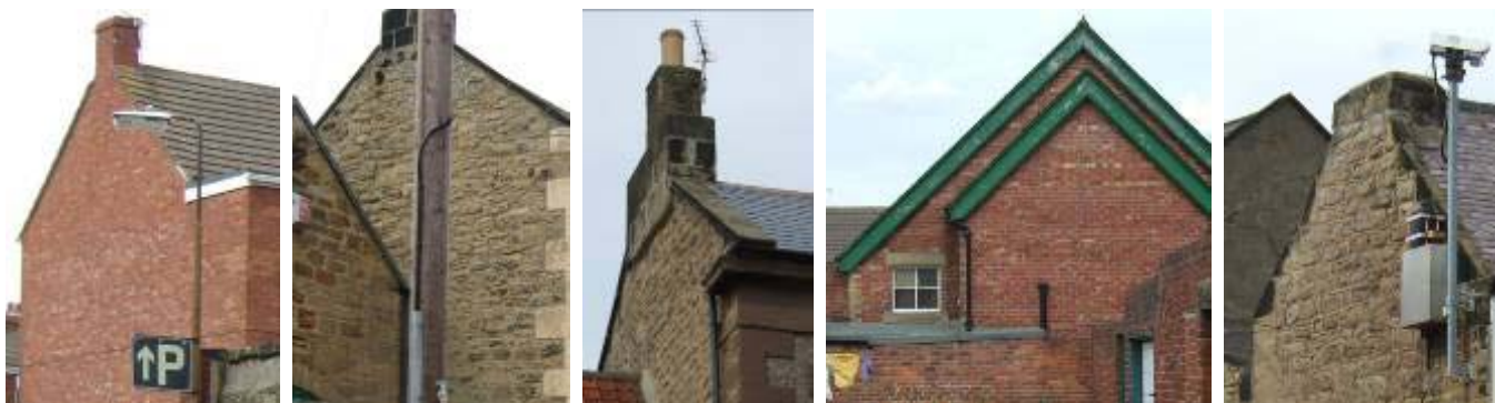
Most verges are plain, some have stone watertabling, some have timber bargeboards. The White House has distinctive triangular stone verge blocks.
