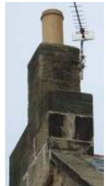
Many chimneys have been removed or are over-pointed or rendered. Some have been rebuilt to smaller proportions.
