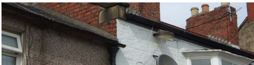
Very few historic cast iron rainwater goods survive, most being poor quality metal or plastic.
