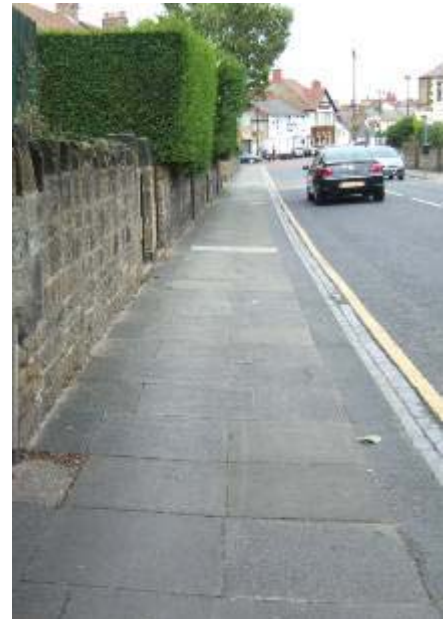
Black tarmac, concrete flags kerbs, scoria block gulleys (far right) and relatively unobtrusive road markings and speed camera.
