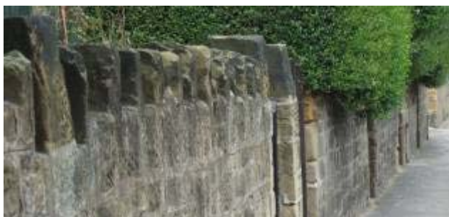
Above: Standing stone wall copes. Below: retaining boundary walls.
