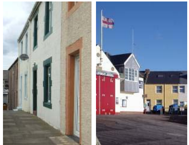
Render can flatten out architectural features. It is sometimes best left unpainted. Whitish tones seem artificial against richly textured sandstone. Modest use of pastel colours and muted, earthy tones can be suitable for this seaside location.
