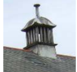
Left: possible remnant fish industry smoke-house roof vent. Below: roof vent to Co-op.
