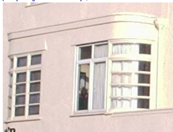
Below: Café Riviera's original curved windows, below, are a key part of its Art Deco style, but its replacement windows, left, are poorly designed 'faceted' bays, not curved.
