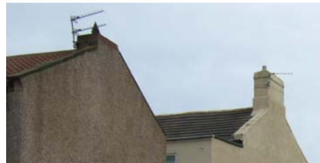
Many chimneys have been removed or are over-pointed or rendered. Some have been rebuilt to smaller proportions.
