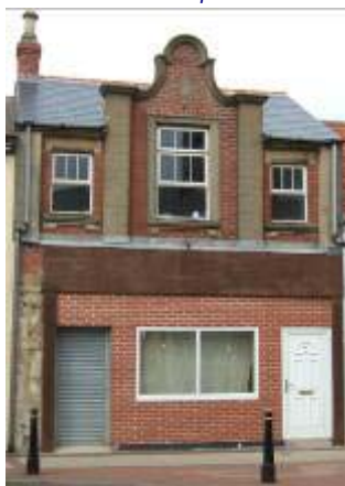
Above: Later additions can harm the appearance of traditional shopfronts. Corbels must be expertly designed and crafted or they will look clumsy against originals. Below: Many shopfronts are altered, with unsympathetic designs and materials, weak detailing, and visual scarring. Bottom: Deep, wide plastic fascia signs unnecessarily dominate the street scene in several places.
