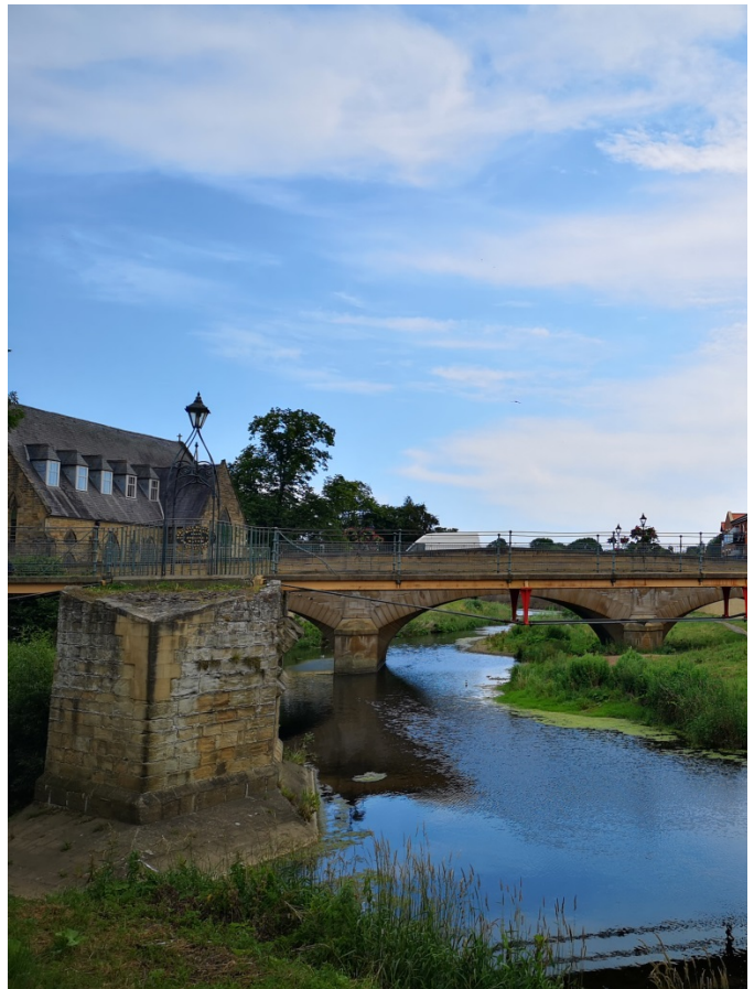
The substantial abutment of the old medieval bridge with decidedly more the dainty footbridge of 1869 on top. In the background we can see the stone arches of Telford Bridge.
