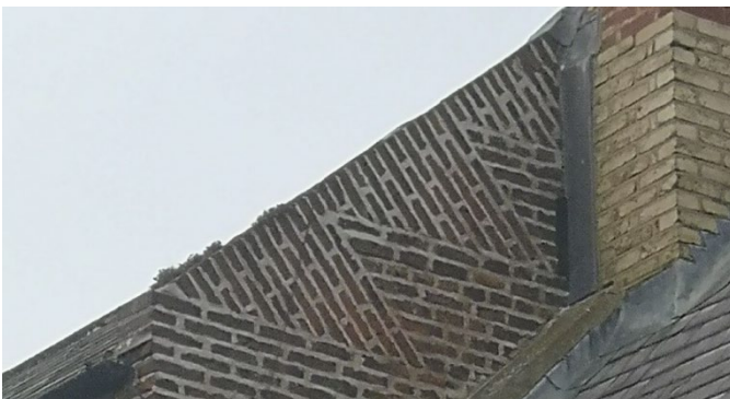
Tumbled in brickwork to gable ends
