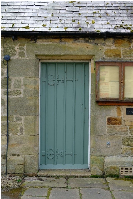
Sneaked rubble walling with distressed lintel and jambs to door. Slate roof. Vertical panelled door with elaborate straps.
