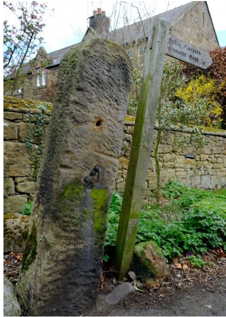
Traditional stone field-gate post, rubble boundary wall.
