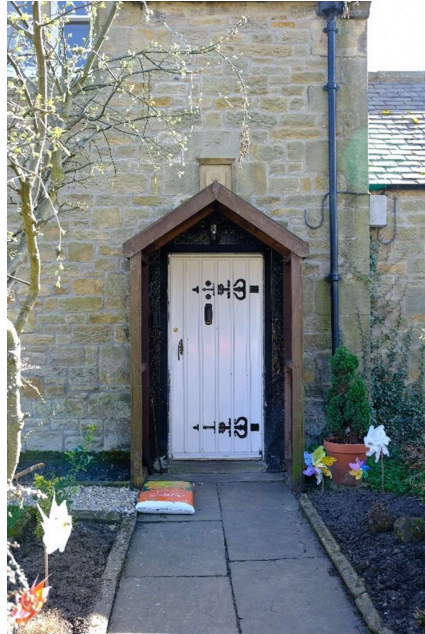
Squared rubble walling with ashlar quoins and inset Percy symbol plaque. Vertical panelled door and ironwork.
