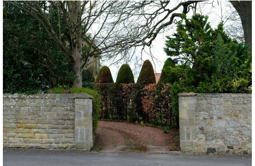
Stone boundary wall with square pins, pyramidal caps and coping. Note different masonry styles to each side of the opening, rock-faced ashlar to left, random rubble to right.
