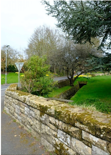
Substantial rock-faced boundary wall and stone retaining walls to Longhoughton Burn.
