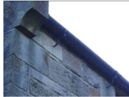
Gutters on spiked brackets, The Green
