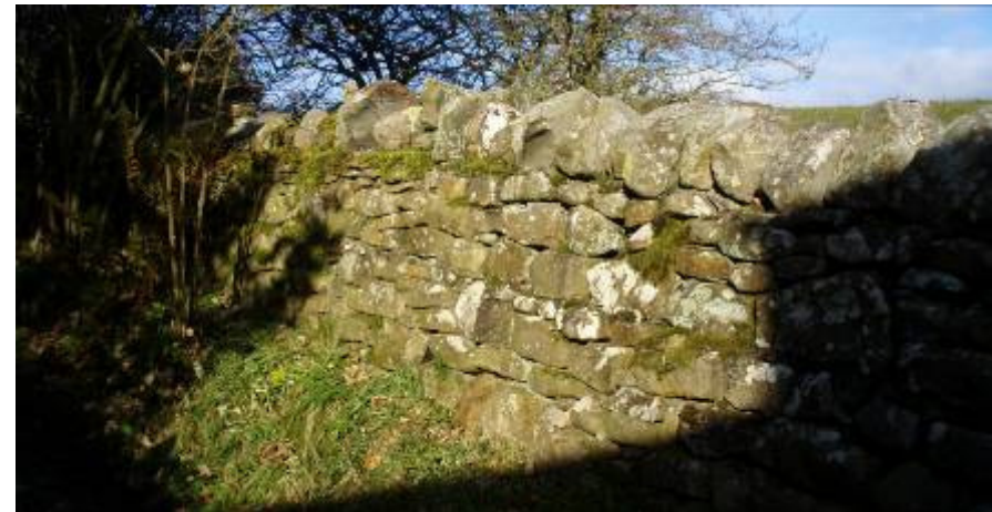
Boundary wall running alongside Whitridge Sike
