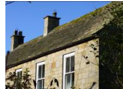
Stone flagged roof, the vicarage
