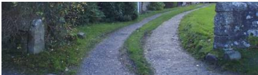
Crushed stone lane on The Green with grass verges
