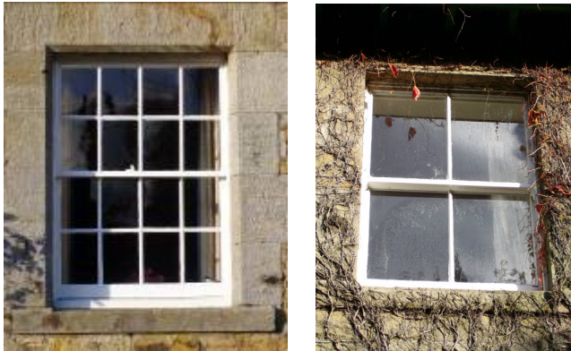
Sixteen pane and four pane timber sliding sash windows in the Old Temperance and Wansbeck House
