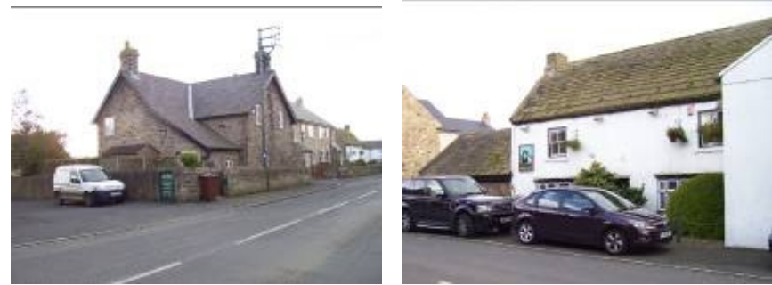
Catslide roof, Castle View House Stone flagged roof, Lion and Lamb
