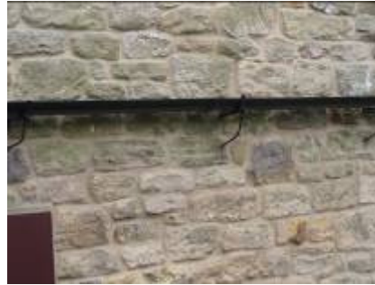
Gutters on spiked brackets
