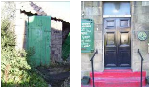
Traditional timber planked and panelled doors are increasingly scarce
