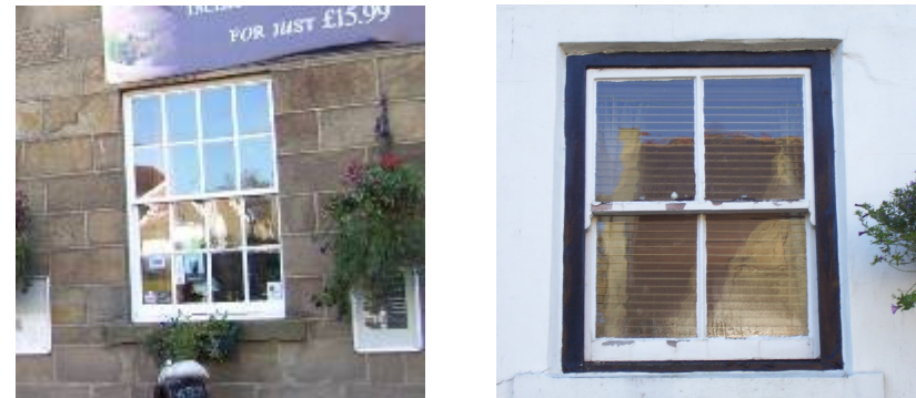
Sixteen pane and four pane timber sliding sash windows in the Crown and Anchor and Lion and Lamb
