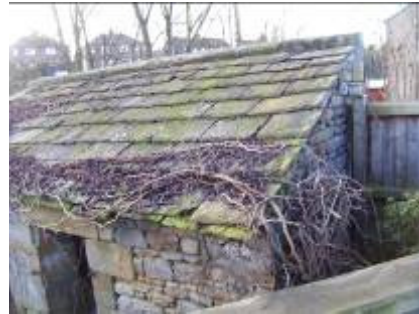
Sandstone flagged roof over an outhouse overlooking Langley Burn
