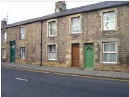
Stone houses & Welsh slate roofs, lower courses showing wear
