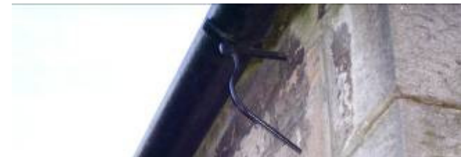
A spiked cast iron gutter, North Bank
