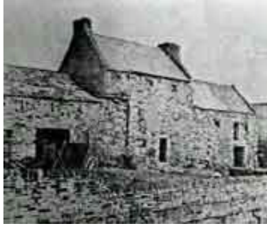
Musgrove Tower before demolition (photograph from www.haltwhistle.org , unattributed)
