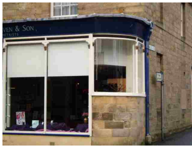
Corner detail - shop front, Westgate
