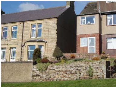
Toothed stone facing at end of terrace, Fair Hill
