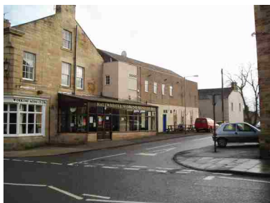
Poor rear extension and badly sited conservatory - Lanty's Lonnen
