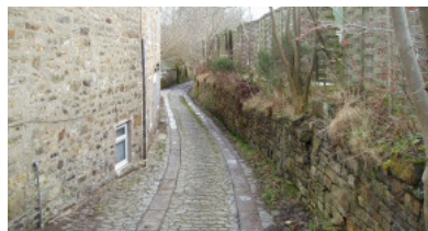
Setts with cart tracks - Mill Lane
