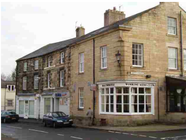
Corner detailing, stone gutter - Working Men's Club, Main Street
