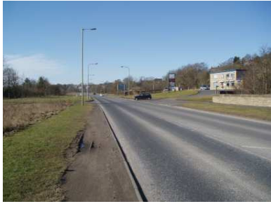
Approach to Conservation area from the east - Avenue St Meen
