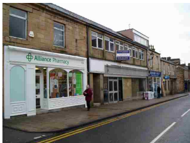
Unsympathetic infill - Westgate. Good modern shopfront at left, but poor replacement windows
