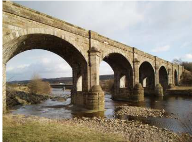
Alston Arches railway viaduct, 1852
