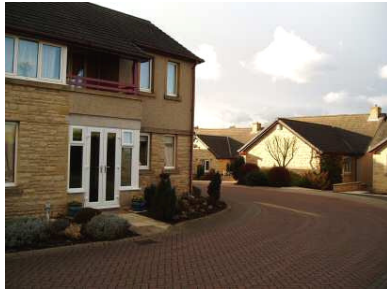
Unsuitable layout, design and detailing - Fairfield
