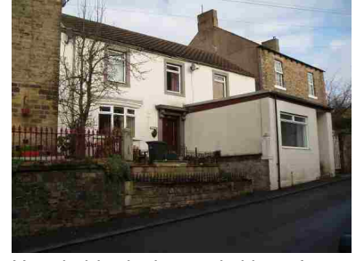
Unsuitable design and siting of extension - Main Street
