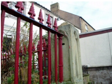
Gothic gatepost and railings - Main Street
