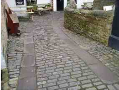
Whinstone setts, with stone cart tracks – southwest corner of Market Square
