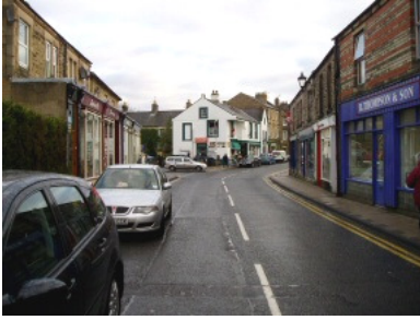
Sandstone, painted render, striped brickwork - Westgate, looking east.
