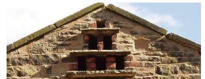
(above) Dovecote in gable end, Churchyard
