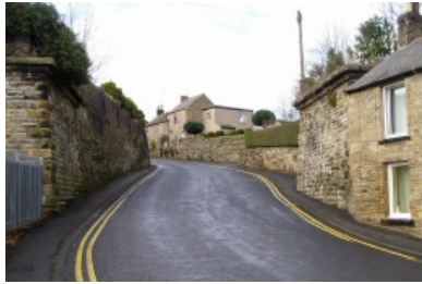
Curved road and retaining walls of the wagonway close the view - Castle Hill, looking west
