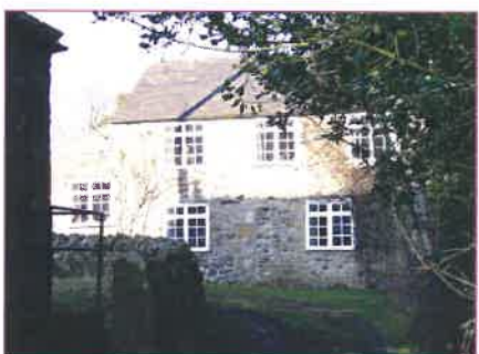
Figure 13 New windows that change the historic character of the south elevation of the terrace
