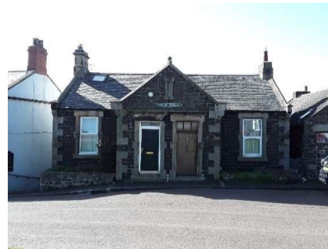
Cottages on Stanley Terrace – architecturally ambitious for their size, incorporating stone quoins, window and door surrounds, finials, kneelers and watertabling and chimneys.
