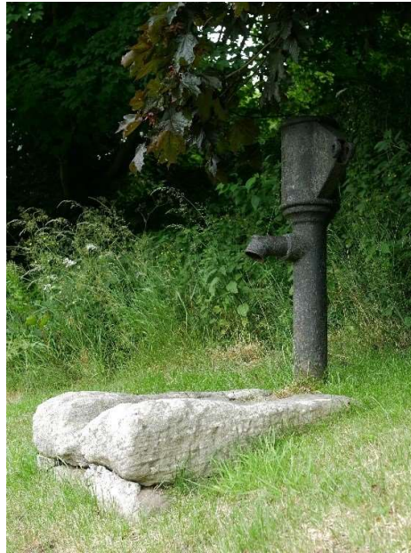
Hand pump and stone block base with drain, Stanley Terrace.
