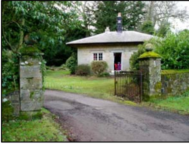
The Lodge, Eglingham Hall
