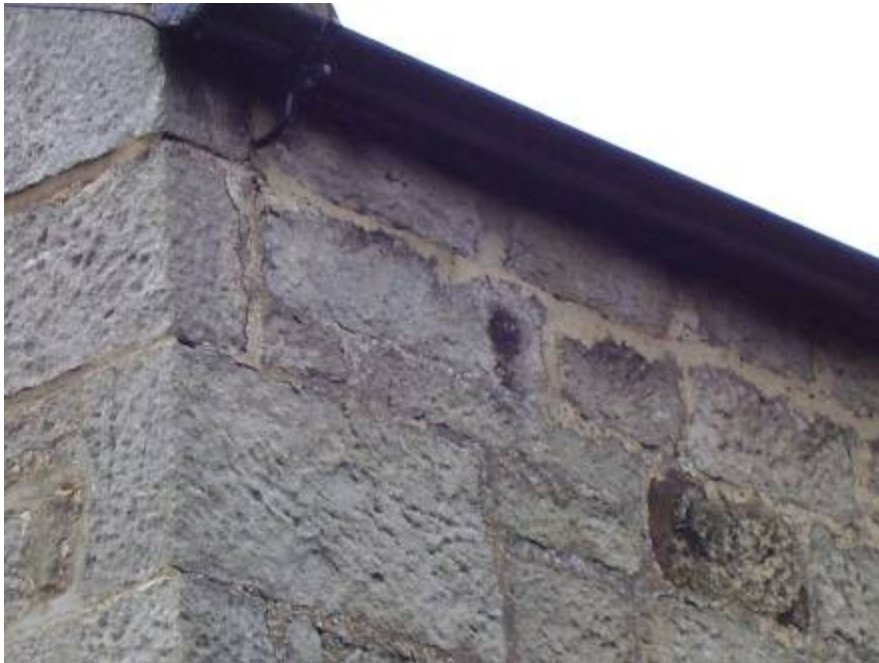
A spiked cast iron gutter, West Farmhouse
