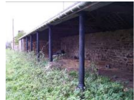
The Hay barn with its distinctive cast iron supports
