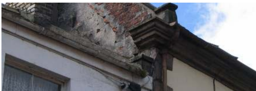
Above left: Plain eaves with minimal overhang. Above right: Decorative eaves with heavy moulded stone cornice. (Both require simple maintenance to clear the gutters to prevent damp)
