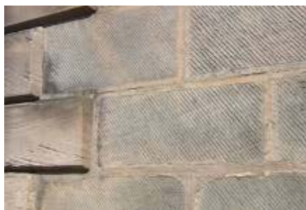
Rough finishing and tooling give considerable texture to the area's masonry
