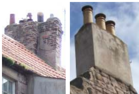
Several chimneys have been lowered, are in poor repair, or have been rendered or over-pointed
