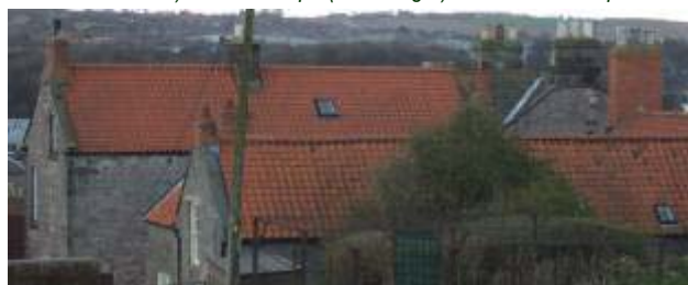
These traditional dual pitched roofs have blank gable-ends (above middle and below) or neater hips (above right). Above left: swept eaves
