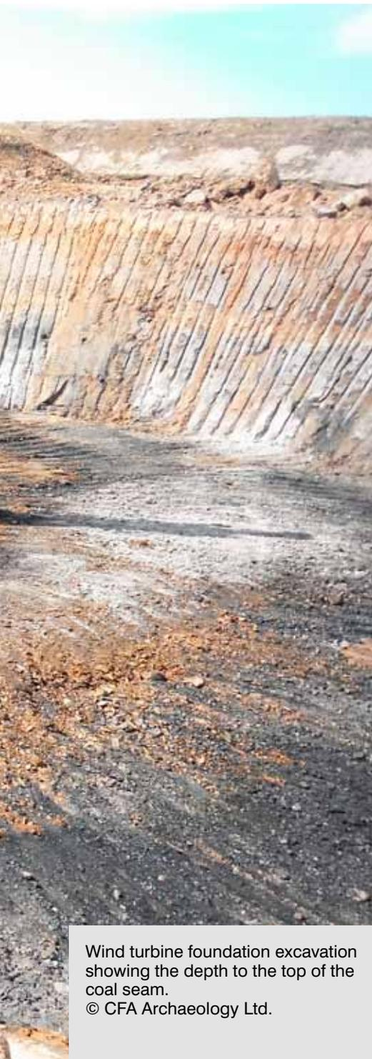
Wind turbine foundation excavation showing the depth to the top of the coal seam.
