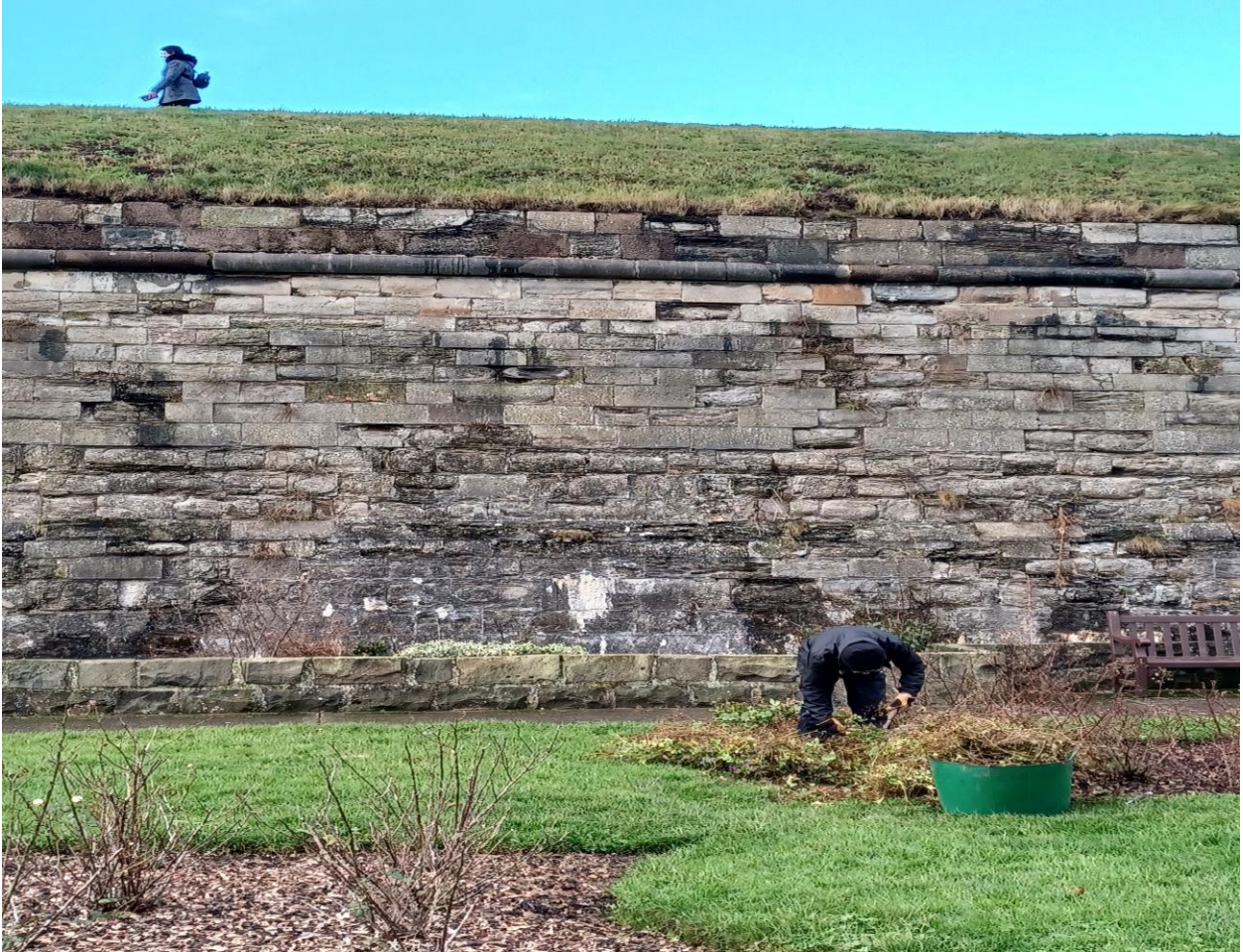
Historic Town Walls & Rose Garden
