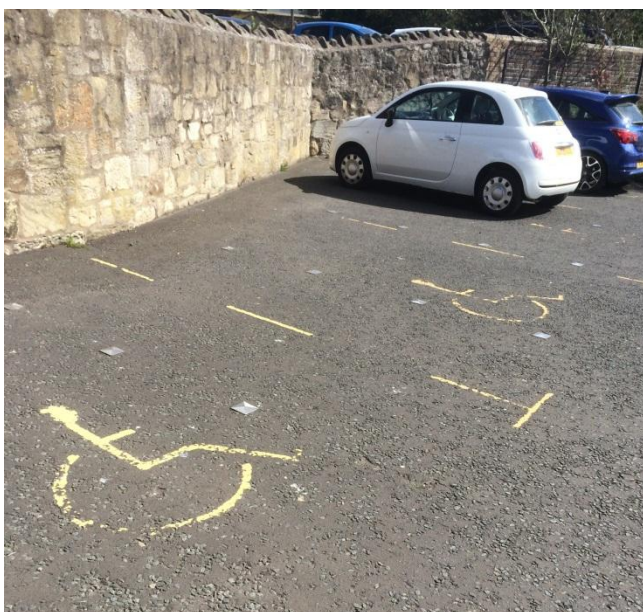
Photo 4: Disabled bay markings not to TSRGD
