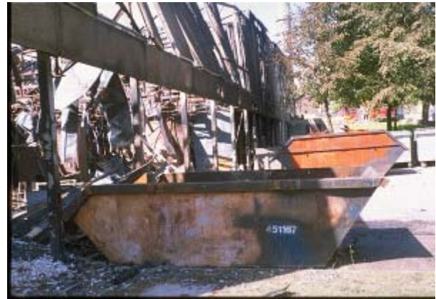
Figure 6 – Damage Caused by an Arson Fire in a Skip
