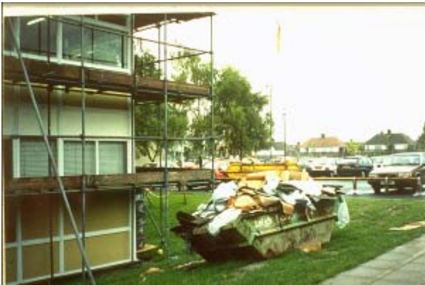
Figure 5 – A Fully Laden Skip Vulnerable to an Arson Attack
