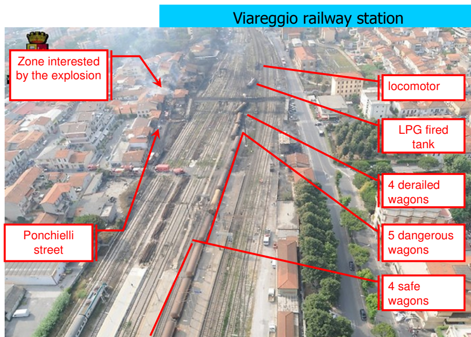
Figure 4.49 – Aerial Photograph of the Explosion at Viareggio Railway Station on 29 th June 2009
