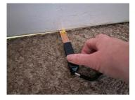
Undercuts of at least 10mm beneath each internal door, to allow air to move through your house. All internal doors that do not currently comply will require this work. The bottom of all 760mm wide internal doors will be sanded down to a gap of 10mm, this does not include external doors.
