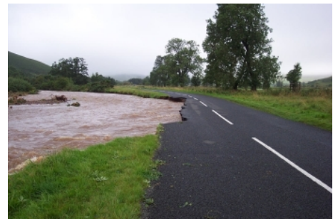
Flood damage at Ingram
