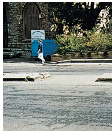
A clear conflict: a refuge intended for pedestrians but unsuitable kerbing opposite.
