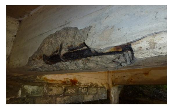
Section loss and corrosion to central main beam at south abutment.
