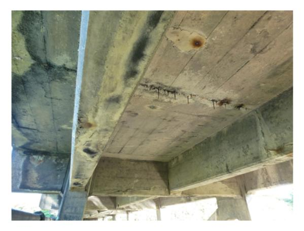
The bridge has been identified as being under strength which is accelerating its decay. At present it is being closely monitored on a regular basis to ensure that it remains safe. This is a significant financial burden.
